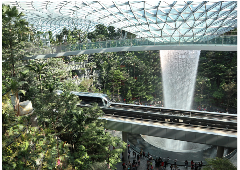
Surbana Jurong was involved in the construction engineering of the Jewel Changi Airport project
