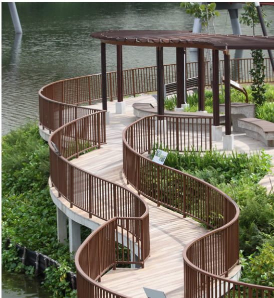
Surbana Jurong designed Punggol Waterway, Singapore’s longest man-made waterway
